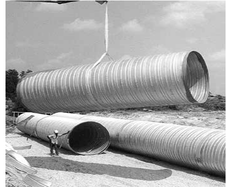
Large Diameter Culvert Pipe
