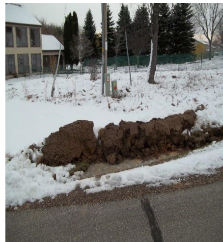
Turf @ Edge of Shoulder Peeled Back
