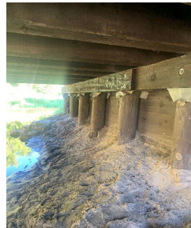
Abutment Cap Replacement Complete
