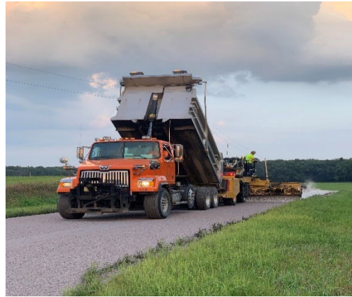
Placing Stone Chips
