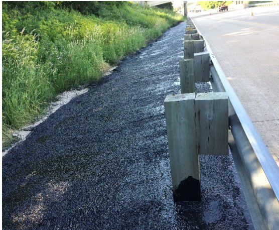
Slope Paving Bank Behind Guardrail
